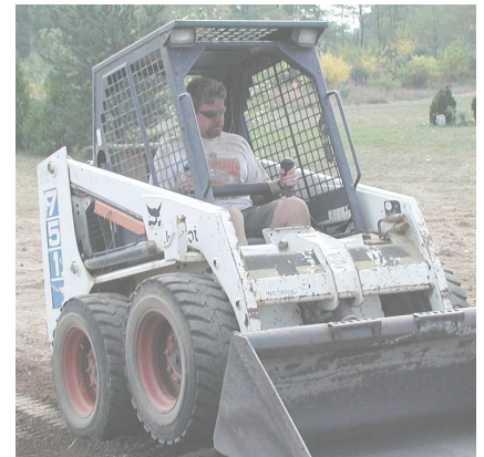
MR. DEAVEN WRECKING A YARD.
